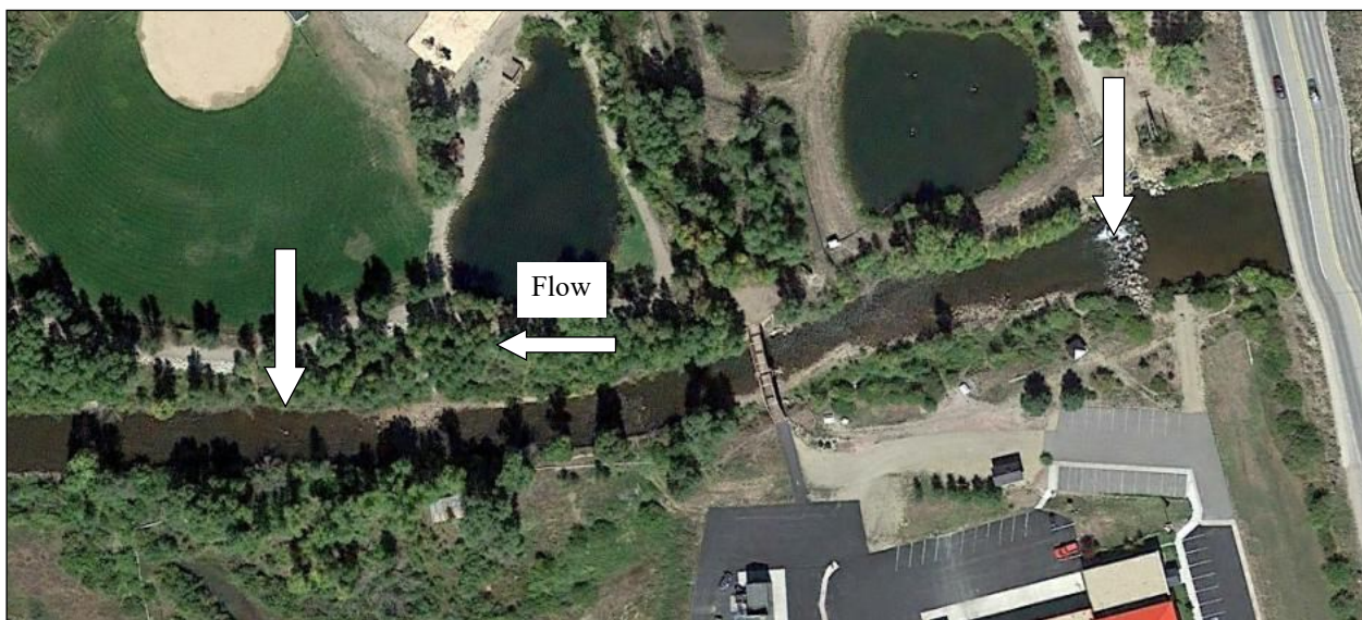
Figure 26. Location of Fraser River Kaibab Park survey station. US Hwy 40 bridge is visible at right.
