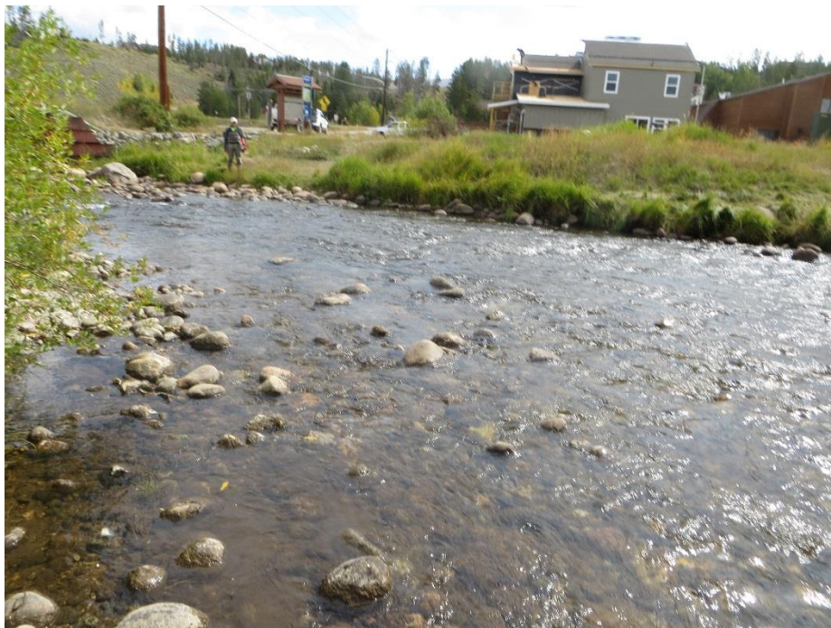
RM STC-0 looking downstream
